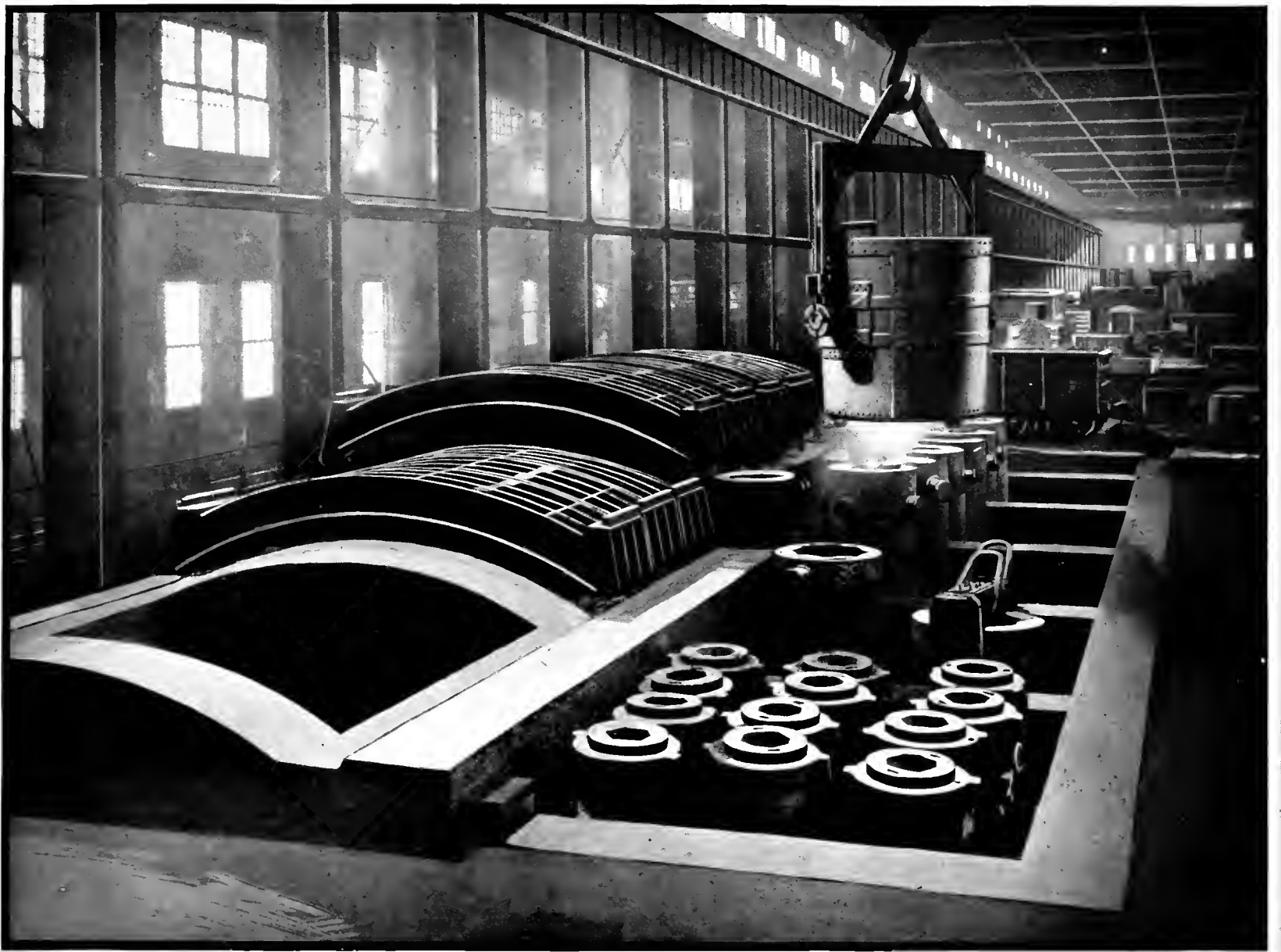
Annealing Furnaces and Ingot Casting Pits
